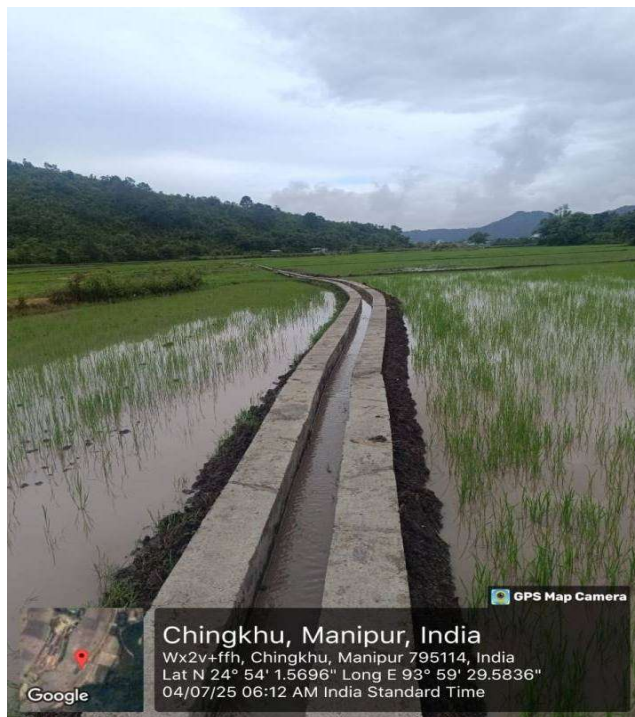
Lined Field Channel under Dolaithabi Barrage Project
