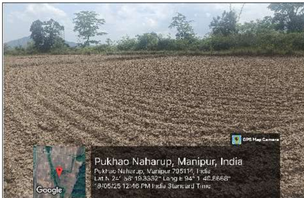
Land Leveling under Dolaithabi Barrage Project
