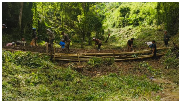
Construction of brushwood check-dam at Hoomi, Ukhrul
