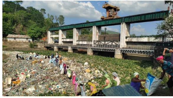
Manipur River cleaning at Ithai Barrage
