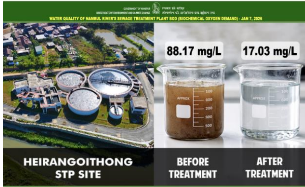
Displaying Water Quality Data for Sewage Treatment Plant (STP) of Nambul River at LED Display Board
