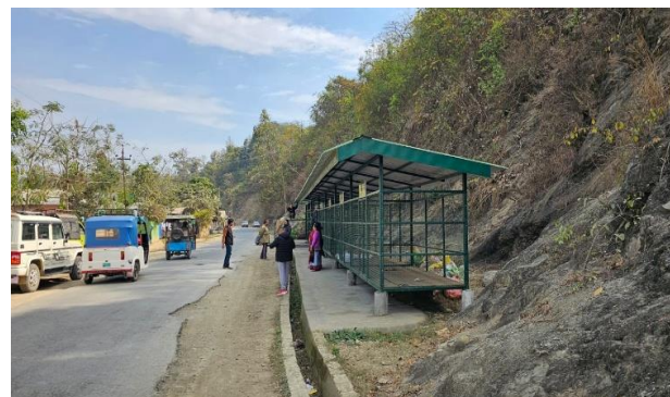
Material Recovery Facility at Sendra
