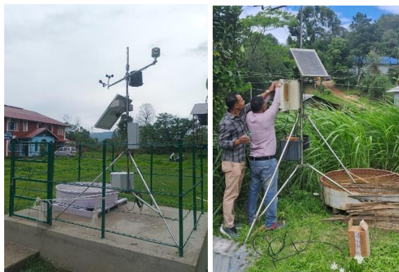
Maintenance and Repairing of AWS
